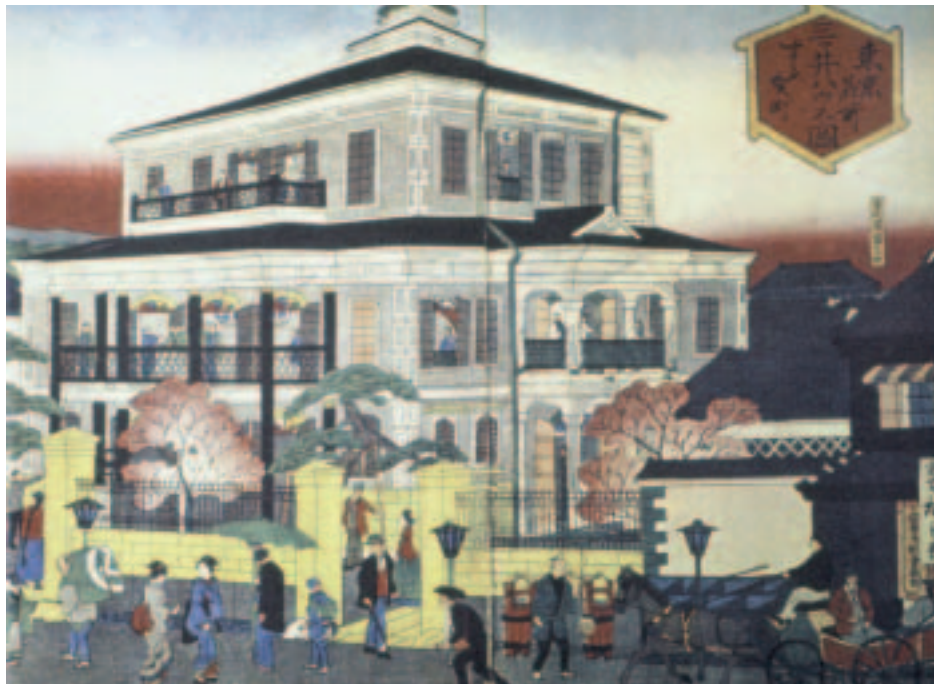
FIGURE 15-27 This 1873 woodblock print of the Mitsui bank is from a series called “Famous Places in Tokyo: Mitsui House in Surugacho” by Ando Hiroshige II or III. The Mitsuis started as merchants, building their family business as the yen replaced rice as the measure of wealth. Would this have been possible in Edo Japan? Why or why not?
